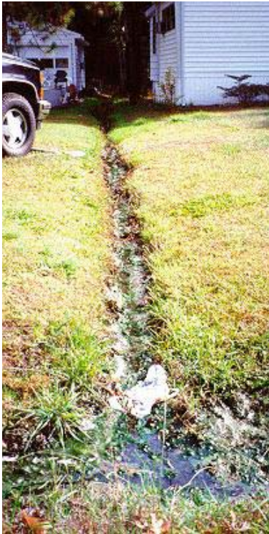
Homeowners whose properties have high water tables are likely to see their traditional septic systems fail quickly. Image courtesy of the Division of Onsite Sewage and Water Services, Virginia.
